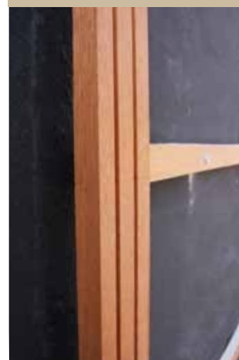
Cutting 1st Plank
